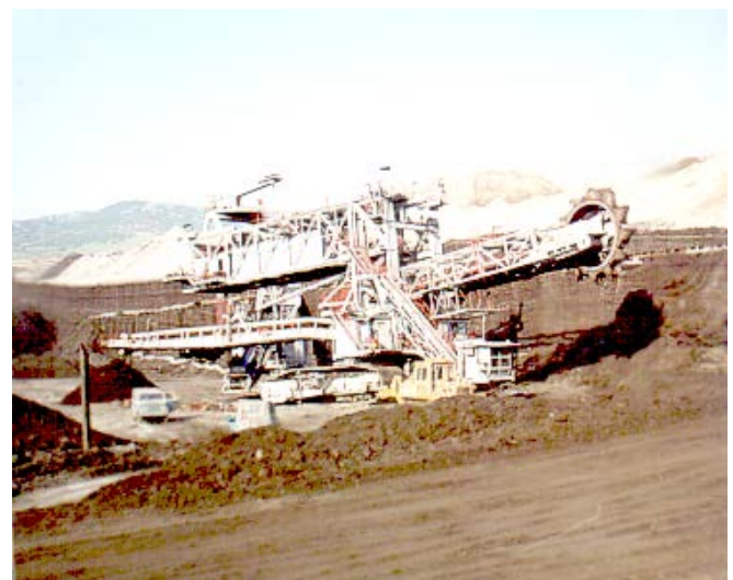
Fig. 4 View of the rotating excavator SRs-630
