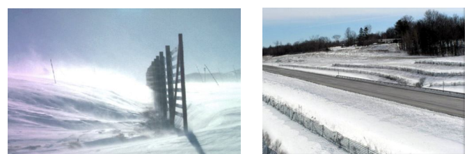
Fig.10 Drift formations leeward the snow fences
