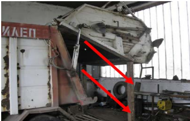
Fig. 8 Primitive substitute for the required special equipment in the mechanical workshop
