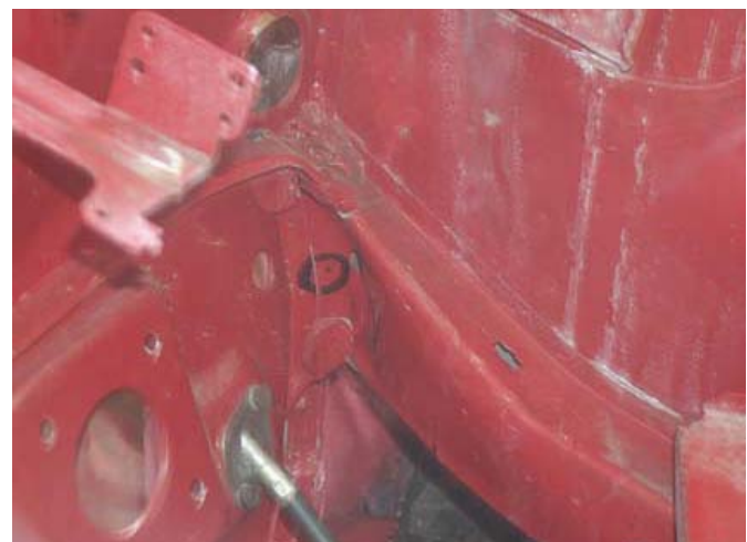
Fig.13 Partition wall after the test
